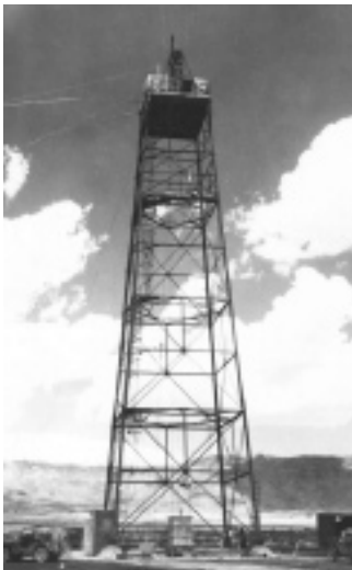
The test tower
